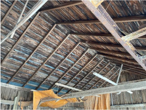
Plate 101: Interior of Outbuilding No. 1 showing rafters and plank sheathing of the roof
