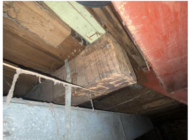
Plate 35: Hand squared floor joist
