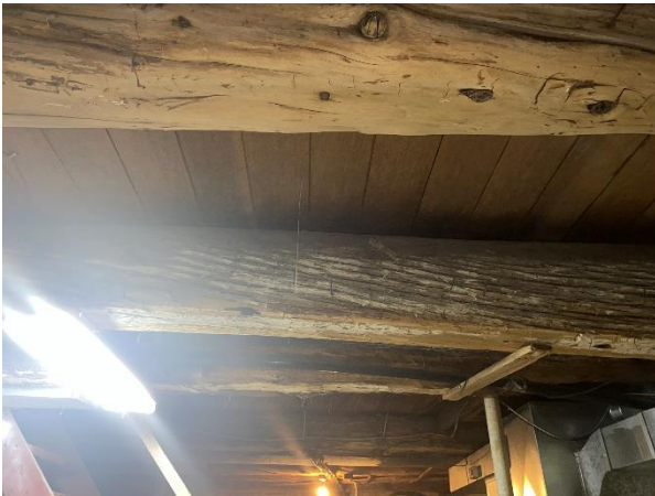
Plate 34: Hand hewn log floor joists
