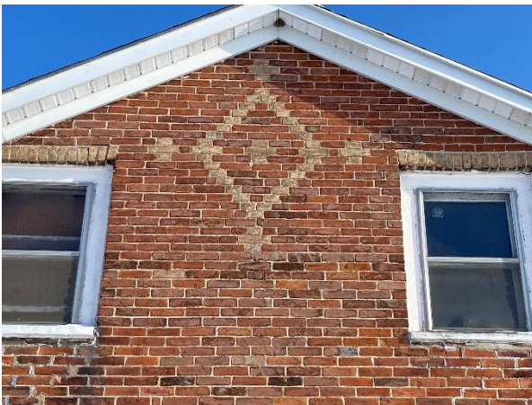
Plate 21: Buff brick diamond and cross pattern
