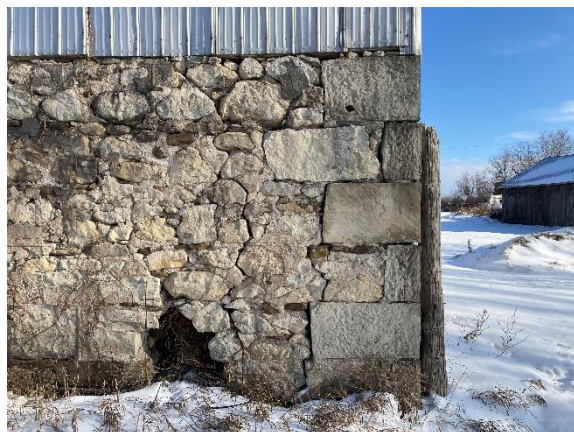
Plate 92: Foundation and cut stone cornerstones of south barn
