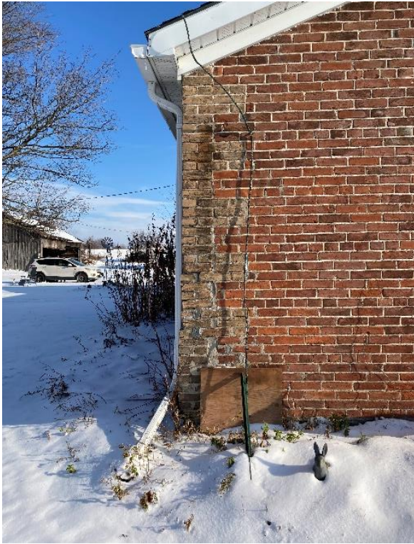
Plate 64: Detail of southwest corner, showing quoins
