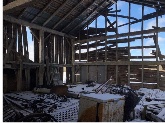
Plate 94: North barn interior showing hand hewn beams
