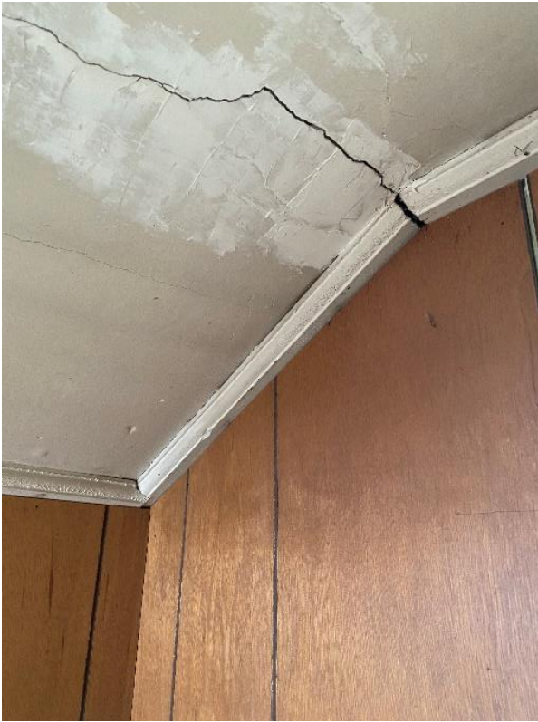
Plate 53: Cracks and repairs of southeast room
