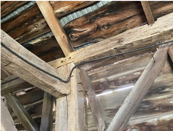
Plate 85: Mortise and tenon timber joints with wood treenails/dowels
