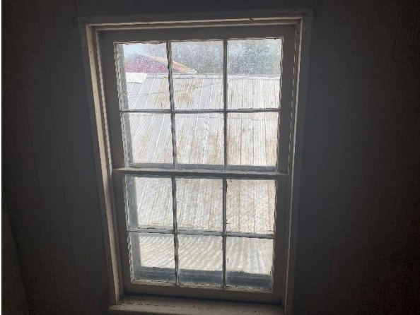
Plate 51: Six-over-six sash window
